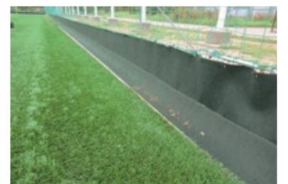
Barrier materials for use in the outer perimeter fences of artificial turf
